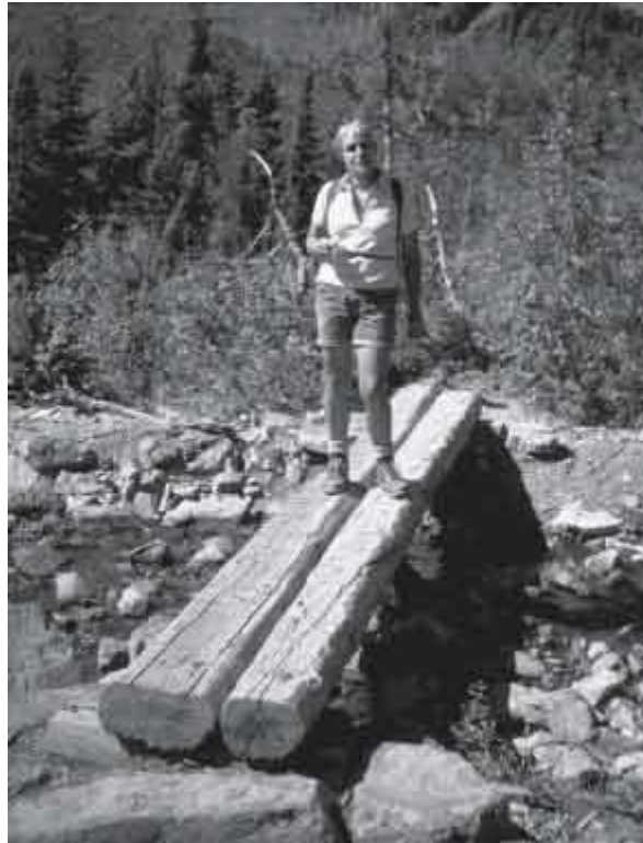
Figure 63--A log footbridge. The sill can be notched to accommodate the logs, but not vice versa. Photo has been digitally altered.
