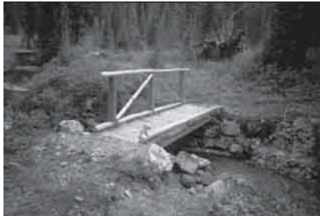
Figure 62--A simple footbridge with a handrail.
