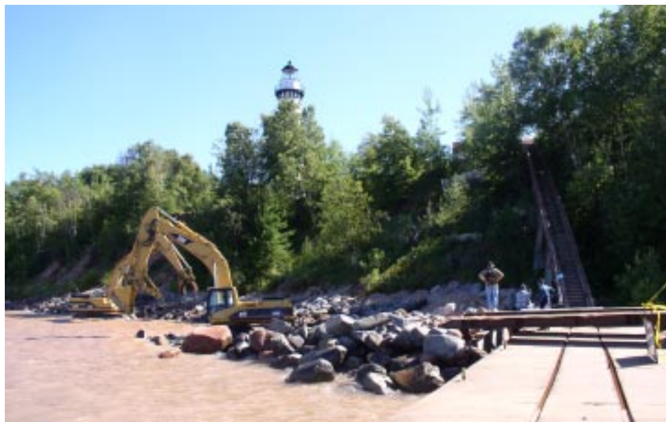
A new rock footing protects the base of the bluff from wave action while a new drainage trench diverts water from the top of the bluff.
