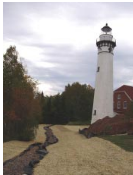
A new rock footing protects the base of the bluff from wave action while a new drainage trench diverts water from the top of the bluff.
