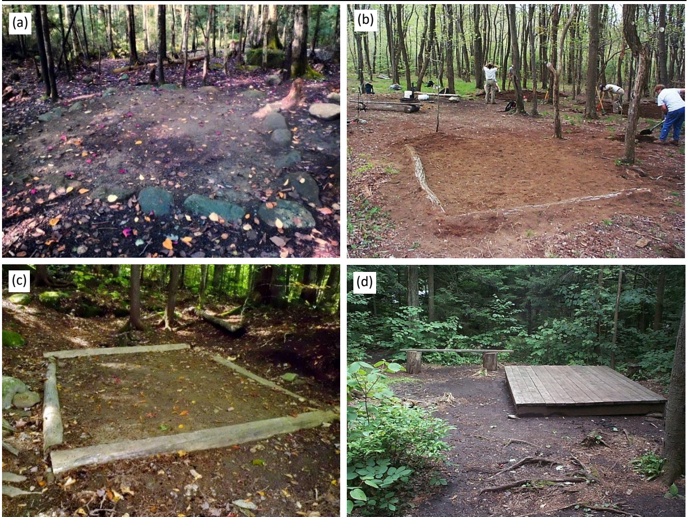
Figure 12. a) Rock-lined tent pad, b) Embedded logs pinned with rebar, c) Wood-lined tent pad, and d) Wood-decked tent platform.
