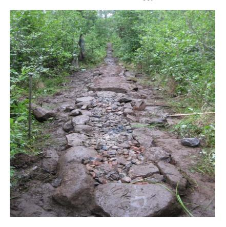
This photo shows a section of causeway before it has been capped with mineral soil. Vegetation is already beginning to shrink the formerly very wide wallow.
