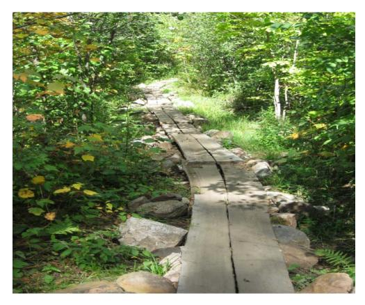
On this boardwalk the planks of one section over- or under-lap the next. Tying them together like this may help keep the boardwalk in place if the site is prone to seasonal flooding.
