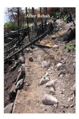
Ogishkemuncie to Kingfisher portage after the Cavity Fire in 2006. The photo on the left shows what the trail looked like shortly after the fire. Rehab crews worked to preserve soils from sliding down the hill by installing rock and log reinforcement. Soil from root wads provided a source for capping.
