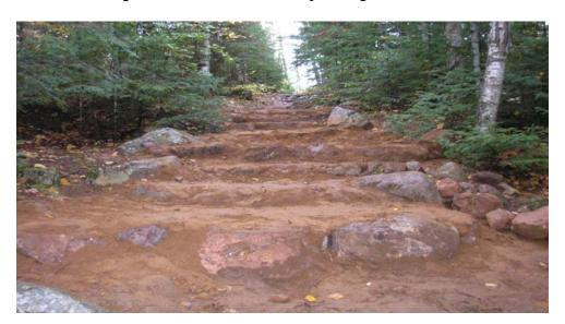
On this slope checks are interspersed with water bars; checks are used in locations where the lay of the land makes it impossible to divert water off the trail.
