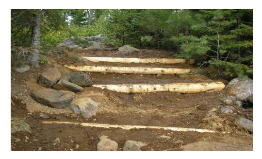
Log checks are built in the same fashion as rock checks. They may be held in place by smaller logs spiked into the notched underside of the check log and buried back into the slope.
